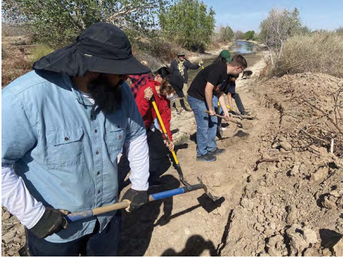
Image 11. Students work alongside volunteers to level out a water channel to allow for more water flow and bank inundation once water is released into the wetlands. Photo Credit: Dr. Ramos-Chavez
