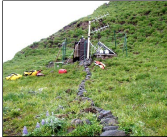
Figure 2.4-17. Pressure Sensor Tide Gauge Station (and Tubing)
